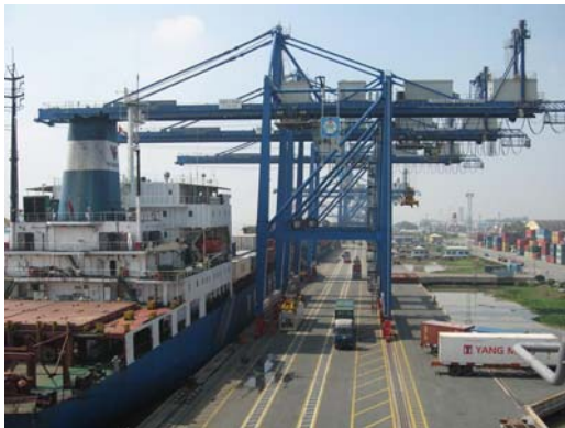
Containerkrane Cat Lai Terminal – Ho Chi Minh City
